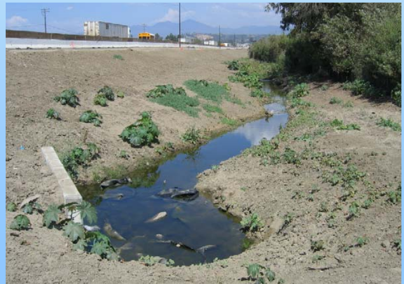
Public agency filled stream channel and lacked BMPs
